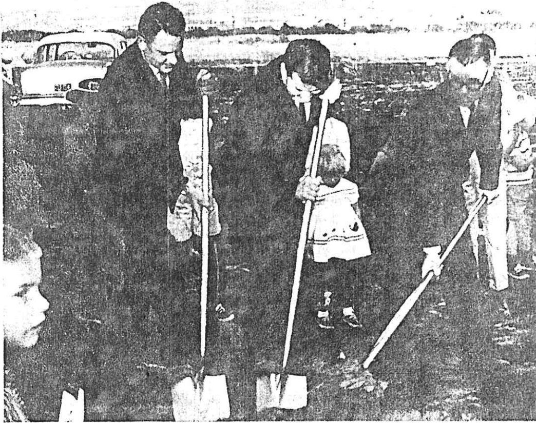
MEMBERS OF THE bishopric of the Idaho Falls 26th LDS Ward bend their backs to turn the first earth to signal beginning of construction of a new $302,000 chapel at 12th St. and Woodruff Ave. Taking part in the groundbreaking are, left to right,
